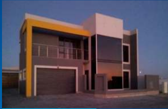
Garage Doors and Windows
